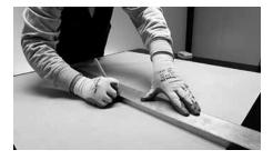
To ensure that scoring is as straight as possible, you may use aluminium levelling rods of the type commonly used by brick layers.
