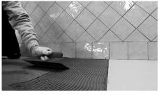
• With a proper notched trowel, immediately follow with a heavier coat of material using the appropriate trowel and enough mortar to provide 100% coverage to the back of the tile and substrate.
